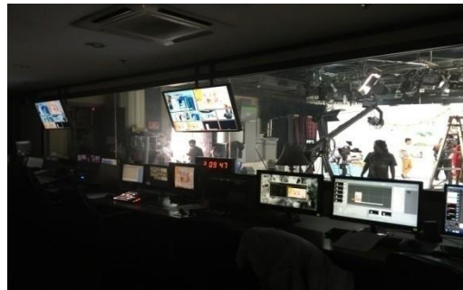
Master Control Room
